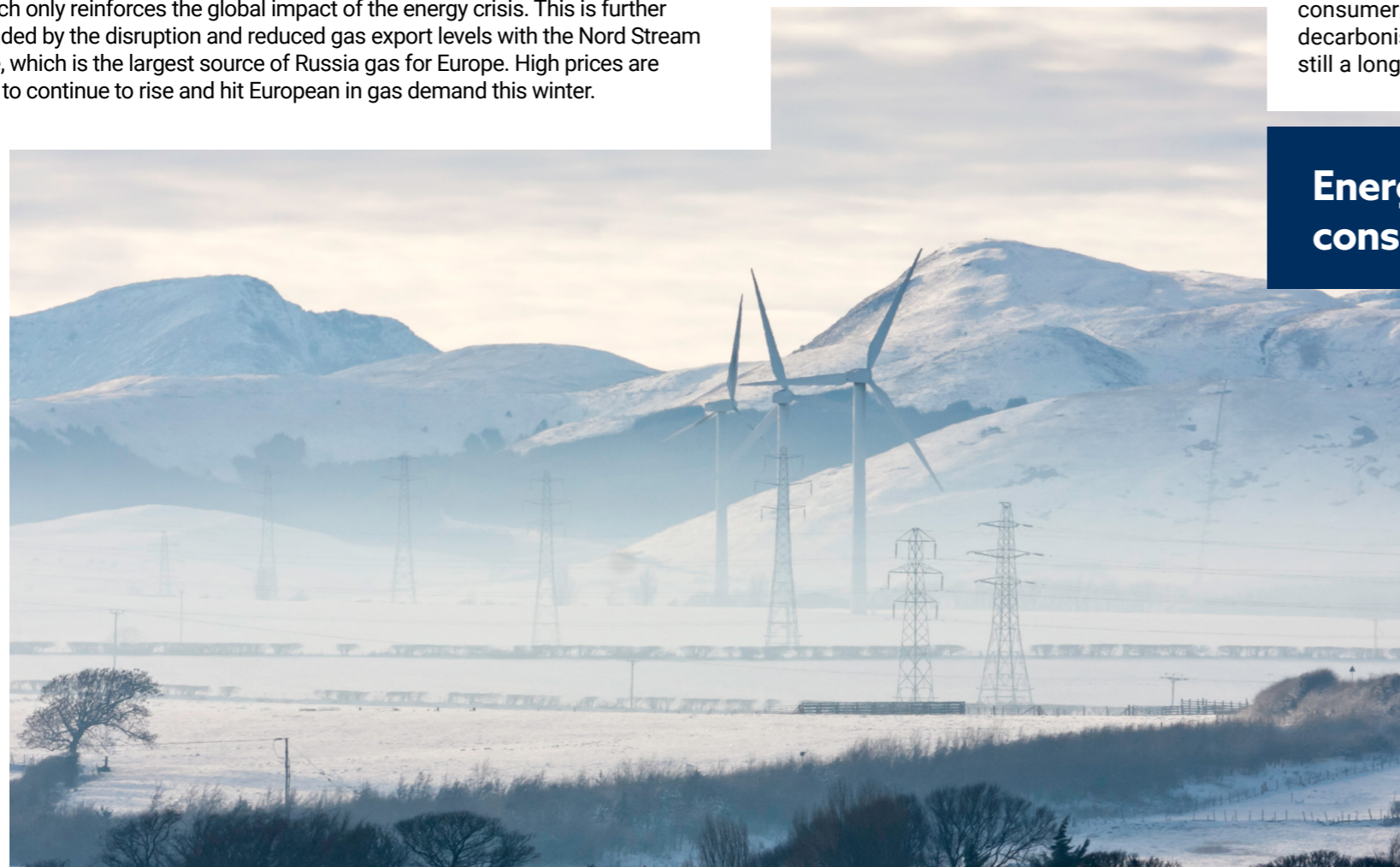
Stainburn wind turbine farm, Cumbria
